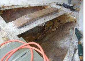
areas I had cut out of the floor. These window frames provided a ledge for the floor sections to rest on for re-installation.
